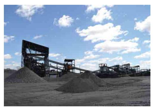
MCM. The coal is extracted from about 80m underground and brought to the surface by a conveyor belt. It arrives (far right) at ground level to be sorted into its different component parts. Some is loaded onto trains for export, while the best quality coal is transported by conveyor belt to Morupule B Power Station
